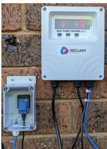
Dry contact wiring between a dry contact switch and controller
